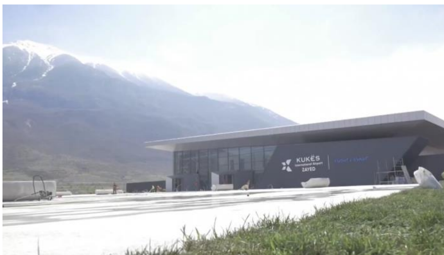
Figure 1.10 Zayed International River Airport in Kukës (Agjencia Telegrafike Shqiptare, 2021b)
